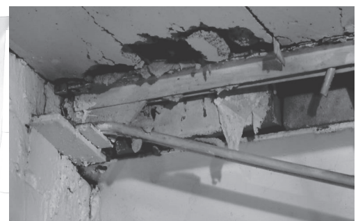
Damaged ceiling from roof leaks.
